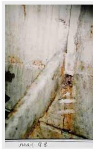
1998 nothing has crossed the top rub off, the stain on the lower rub off has almost faded away, proving it is no longer being fed (the tear of a dying rust cell).
