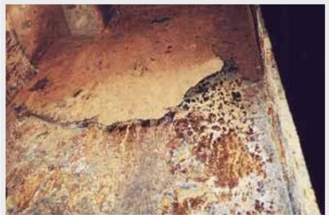
Looking up, the bulk head above shows a large sheet of original hard coating disbonded and hanging.
