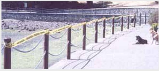
These posts get direct spray from the ocean causing rusting at grade and below. Our objective is to stop the rusting and prevent future rusting.
