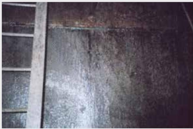
This area had been submerged in waste water for approximately four months, from August to the end of December 2002, when they finally got pumped out and hosed down. But now there is no rusting here, the **Ship-2-Shore** coating is 100% intact.
