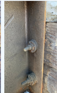
Steep Creek Bridge - 18 yrs after application of S2S
