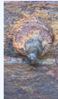
Steep Creek Bridge - Uncoated
