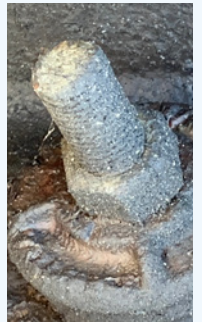
Steep Creek Bridge - 18 yrs after application of S2S
